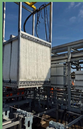
Figure 1 – ZeeLung-kassette under installation i anoxisk tank
